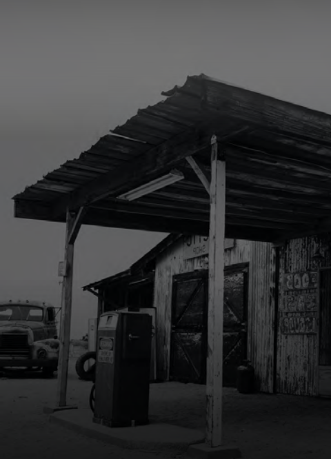
LACK OF CHARGING INFRASTRUCTURE
